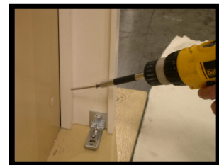
With PIVOT Leg Straight and LEVEL, screw Leg to the Wall
