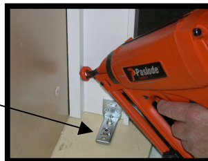
With PIVOT Leg Straight and LEVEL , Nail Leg to the Wall
