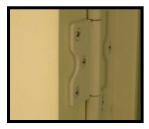
Hinge spacer installed
