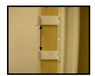
Tip: For flush panel installation, line the backside of hinge barrel with the wall surface.
