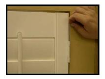
10. Check gaps between panels and around the window opening; adjust accordingly. Ideally panels should rest lightly on the sill whenever possible.
