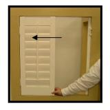
9. With all hinge pins installed, open the left panel and place the right shutter panel into the window opening and slide into position. Once panel is aligned with frame hinge, insert hinge pins into all hinges to secure the panel.
