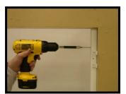
With hinge aligned, secure the top screw.
