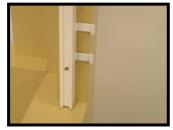
Once top screw is tightened, line up the bottom hinge in reference to top hinge position.
