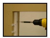
With hinge aligned, secure the top screw.
