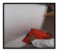
Note: After ensuring that your center stiles and side boxout are aligned, you can go back and add additional nails/screws to completely secure your boxout frame.
