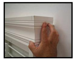
13. Fill nail/screw holes and caulk sides if necessary.
